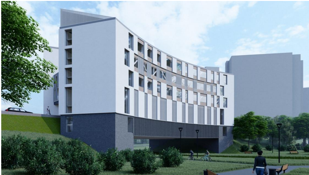
Figure 7. Model of a hotel and residential BB on the site of the Igarsky bridge in the Sviblovo district. Moscow. Architect A.M. Andrienko
