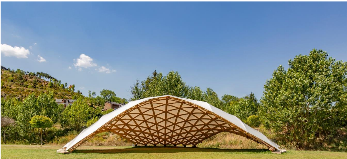
Figure 5. Main view of the timber structure which has a PVC cover and has two layers of wood in different directions. Thanks to the double curvature it was possible to obtain much greater rigidity and resistance. Source: Andrés Flajszer
