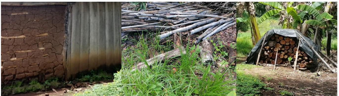
Figure 3. Photos of the house
